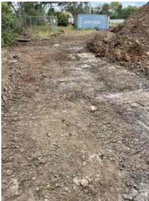
Photograph 3 – Removal area subsequent to remediation works
