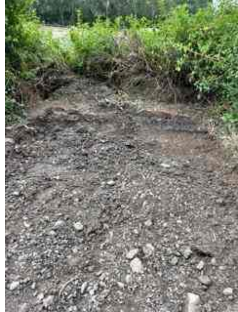
Photograph 2 – Removal area subsequent to remediation works
