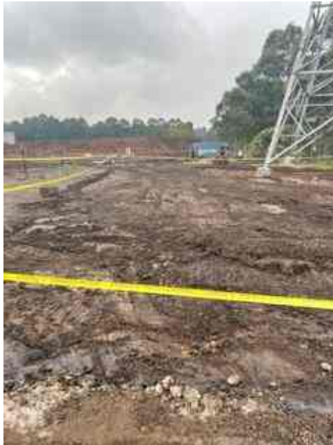
Photograph 1 – Removal area subsequent to remediation works
