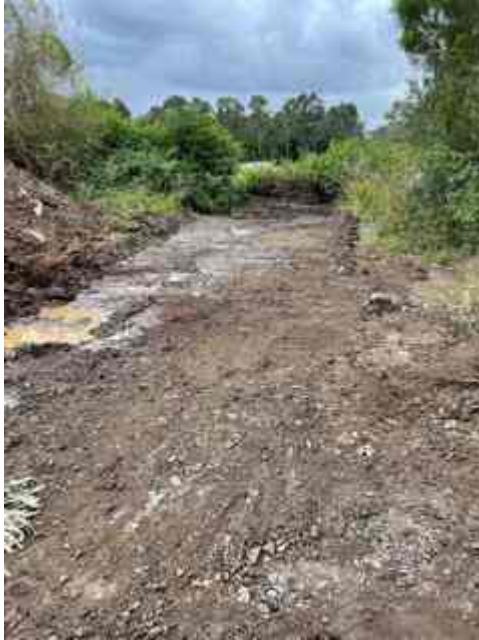
Photograph 1 – Removal area subsequent to remediation works
