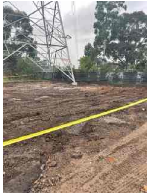
Photograph 2 – Removal area subsequent to remediation works
