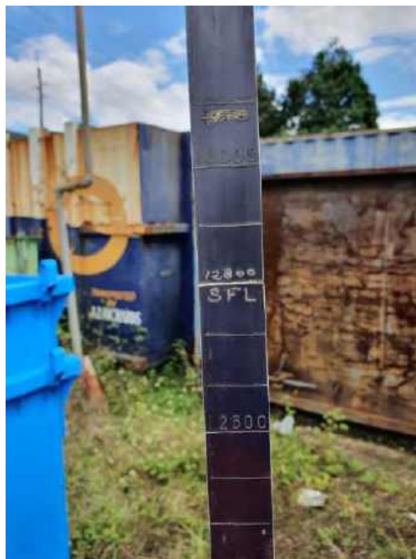
PHOTOGRAPH 6 Dip stick of 13,000L UPST, with vent in background.
