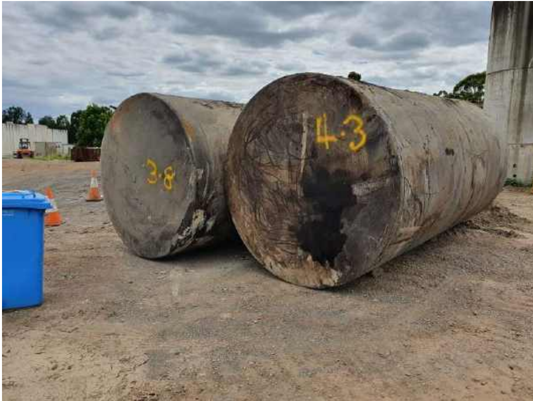
PHOTOGRAPH 7 Condition of removed Tanks 1 & 2.
