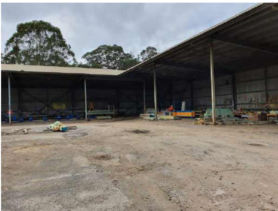
PHOTOGRAPH 2 View east of L shaped open building.
