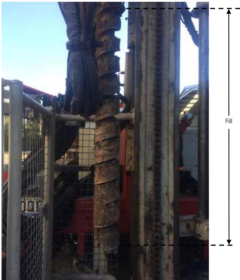
Photo 1: Retrieval of fill materials (from ground surface to a depth approximately 1.5 m) from the auger at BH503 (viewing east).
