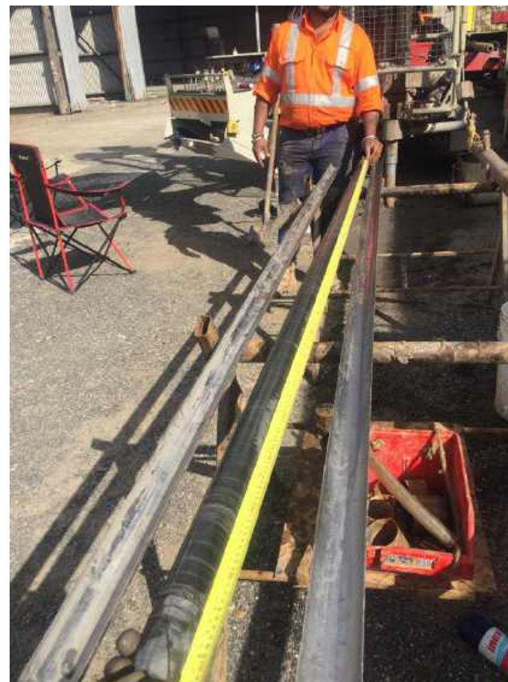
Photo 4: Retrieval of rock core (depth approximately 2.3 m to 5.08 m) from BH502 (viewing northwest).
