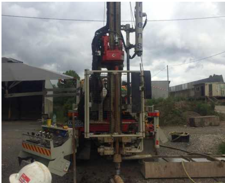
Photo 3: Progress of rock coring at BH501 (viewing west).
