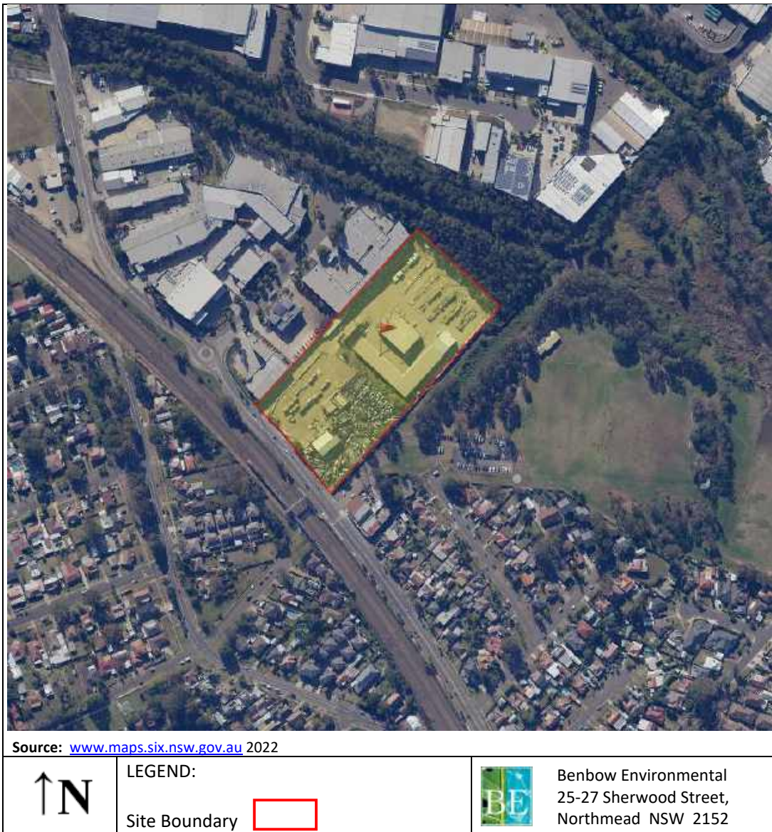
Figure 2-2: Aerial Photograph of the Site and Surrounds
