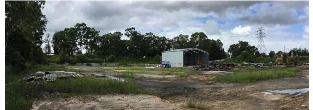
9 View south-east across the site.
