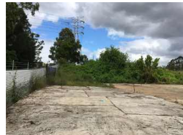
14 South-eastern corner of the site.
